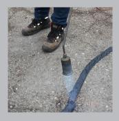
Sufficient heat has been applied when the material starts to bubble.
