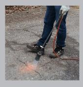
Brush away any dirt and remove moisture from the crack with a heat torch
