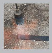
Bond BandFill to the crack by heating the material with beat torch
