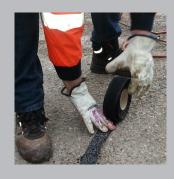
Roll BandFill onto the surface following the path of the crack
